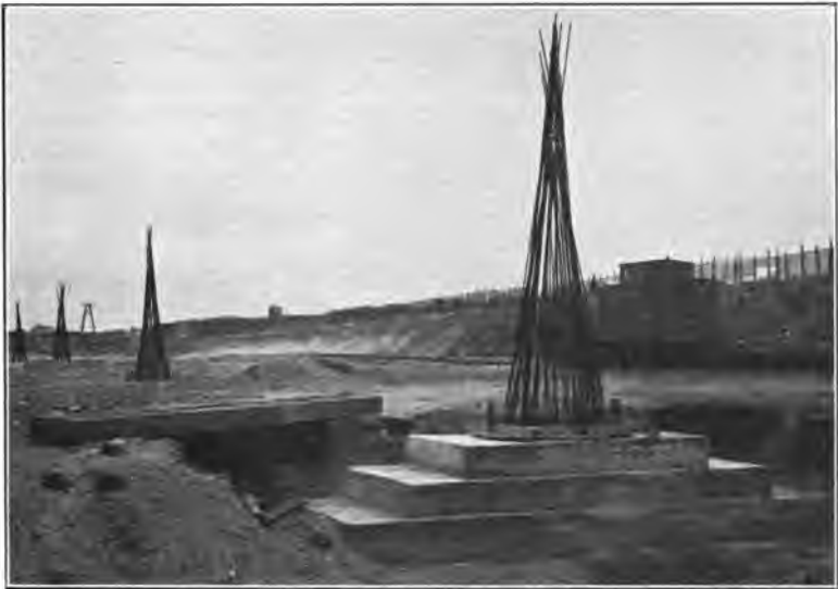
FIGURE 1 CONCRETE BASE AND RE-ENFORCING FOR COLUMNS
